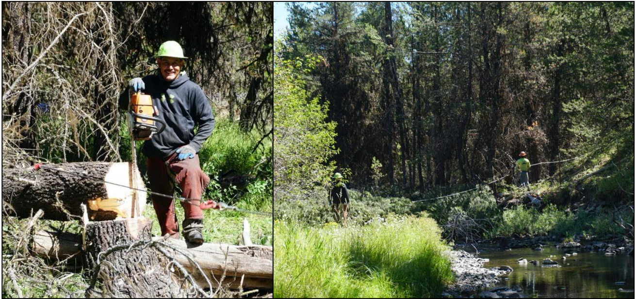
Photo 5: Setting up the grip hoist cable to build a large woody debris jam on Camas Creek.
