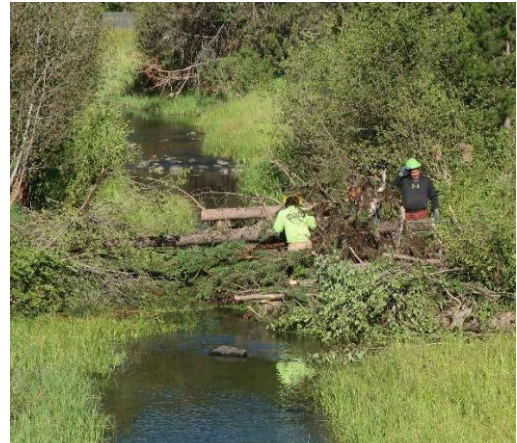
Photo 2: Crew building lateral deflector LWD structure on Camas Creek.
